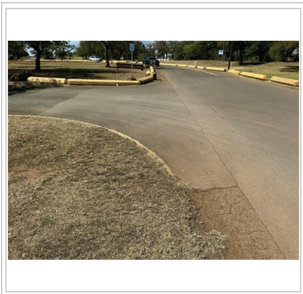
Area to be repaved
