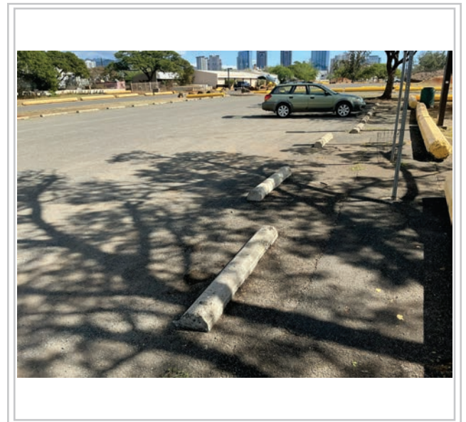
Area to be repaved
