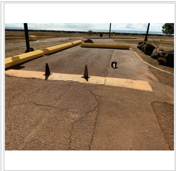
Area to be repaved
