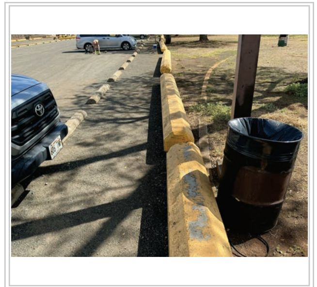
Area to be repaved
