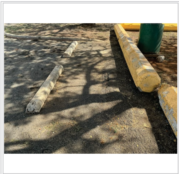
Area to be repaved
