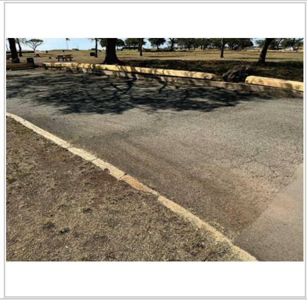
Area to be repaved
