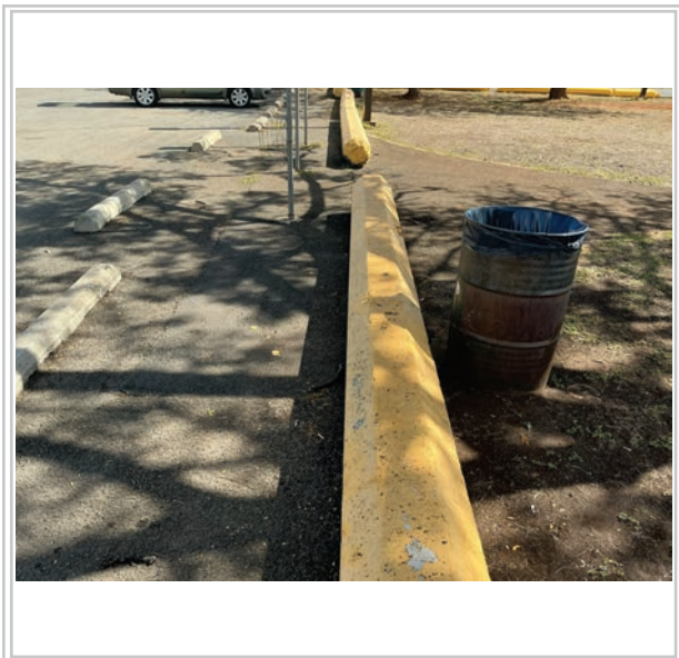
Area to be repaved
