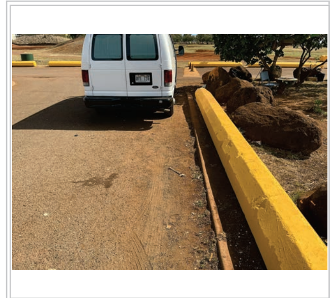
Area to be repaved
