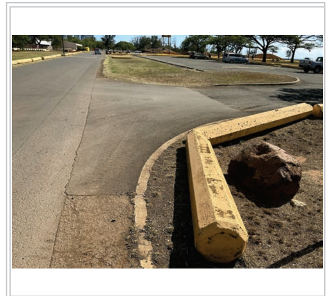
Area to be repaved
