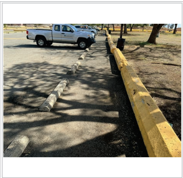
Area to be repaved
