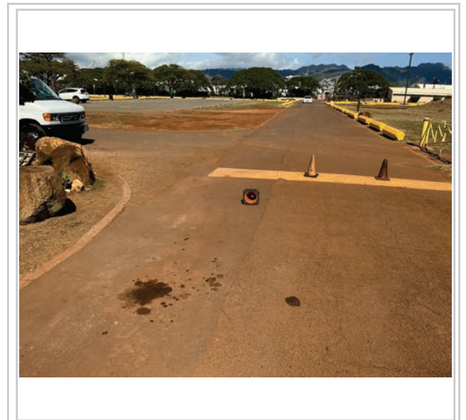
Area to be repaved
