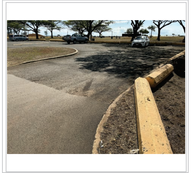
Area to be repaved
