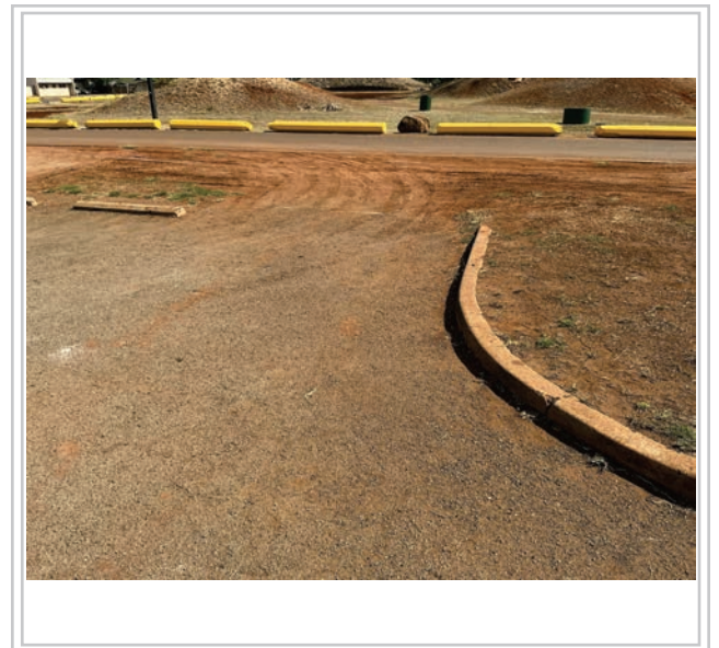
Area to be repaved
